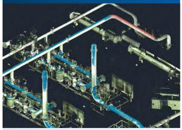
Generate on-demand, accurate as-built data for building design and retrofit projects. With more precise and comprehensive data, you can ensure the design will work. You can also validate the design by comparing the virtual overlay and the as-built data of the site to perform clearance checks and clash detection.
